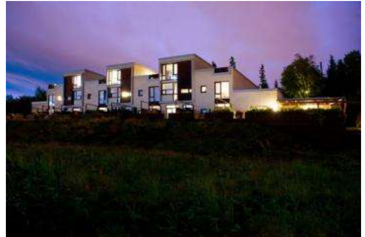
Terraced Housing - Norway ROJO Architects High Insulation Levels; Ground Sourced Heat Pumps; Heat Recovery Ventilation. Photo: Elisabeth Lund
